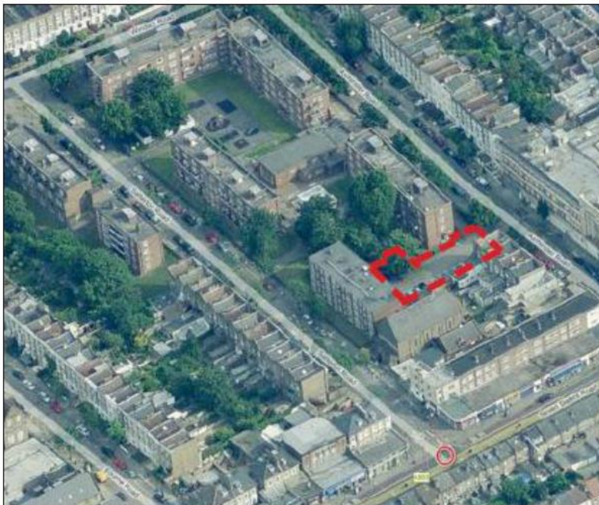
Photo 1 The site looking north east
