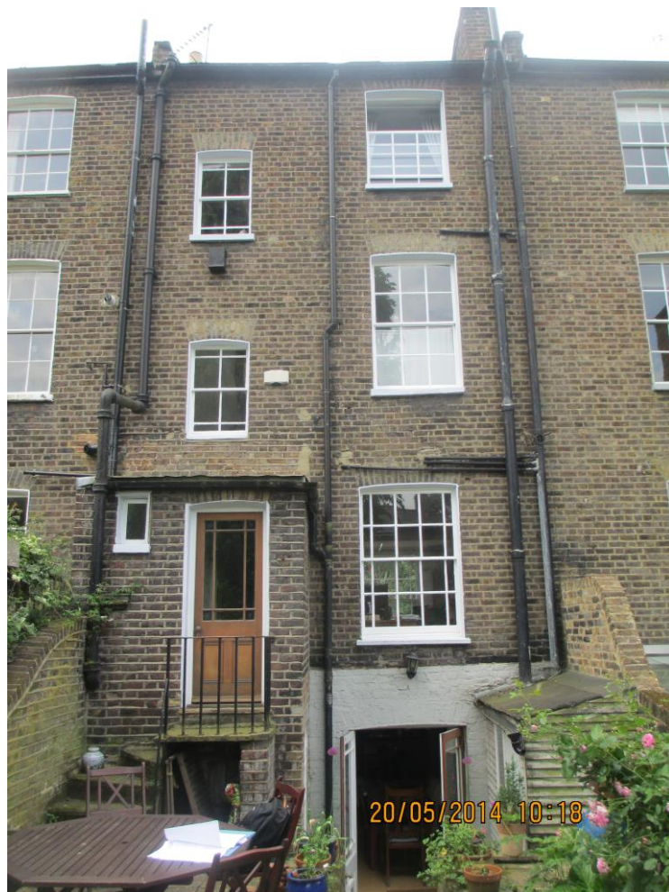
Image 2 - View of rear elevation of the site
