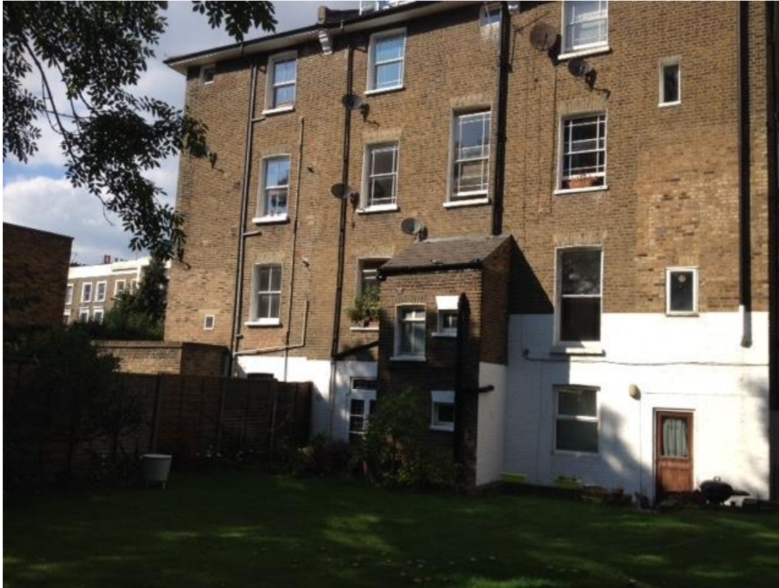
Photo 1: View of rear elevation and part of rear garden
